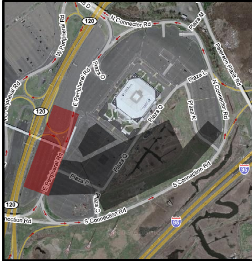
Figure 2: Aerial Photo of Complex Site Previous to Construction
